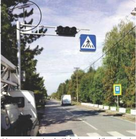
Pedestrian crossing signal with lantern and three illuminated running pedestrian figures powered by solar panels
