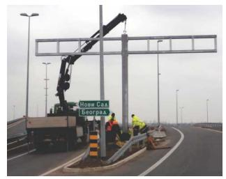
Cantilever production and installation
